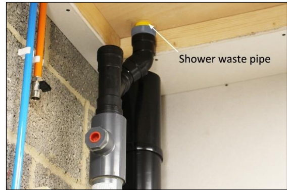
21. Connect the open end of the second 45° connector (Item 5) onto the reducer attached to the shower waste pipe.
