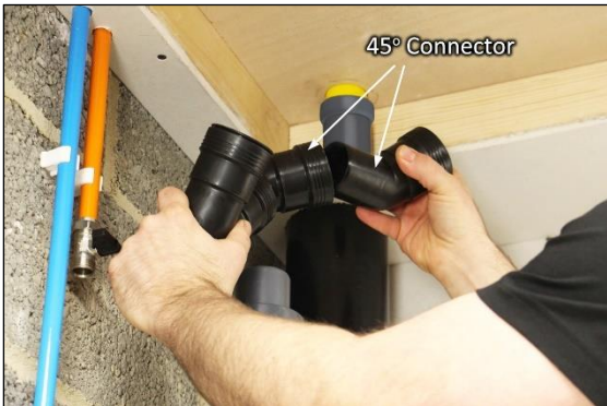
20. Insert the second 45° connector (Item 5) into the end of the other.
