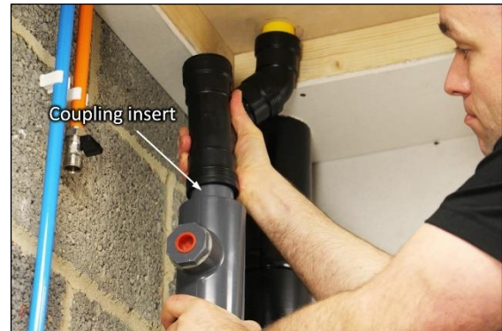
22. Connect the bottom of the T-piece (Item 3) onto the top of the Pipe+ HE and the coupling insert (Item 2).
