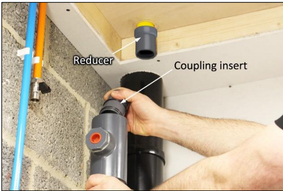
17. Push a coupling insert (Item 2) into the top of the Pipe+ HE.
