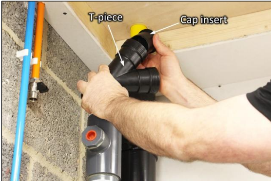
18. Push the Cap insert (Item 4) into the top of the straight section of the T-piece (Item 3). The straight position must not be used to connect to the shower waste pipe.
