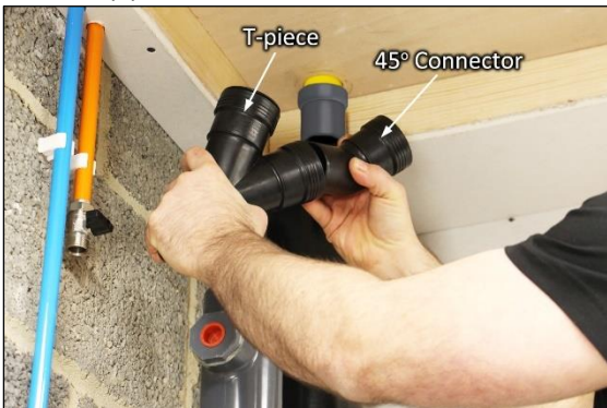
19. Insert one of the 45° connectors (Item 5) into the 45° opening of the T-piece (Item 3).
